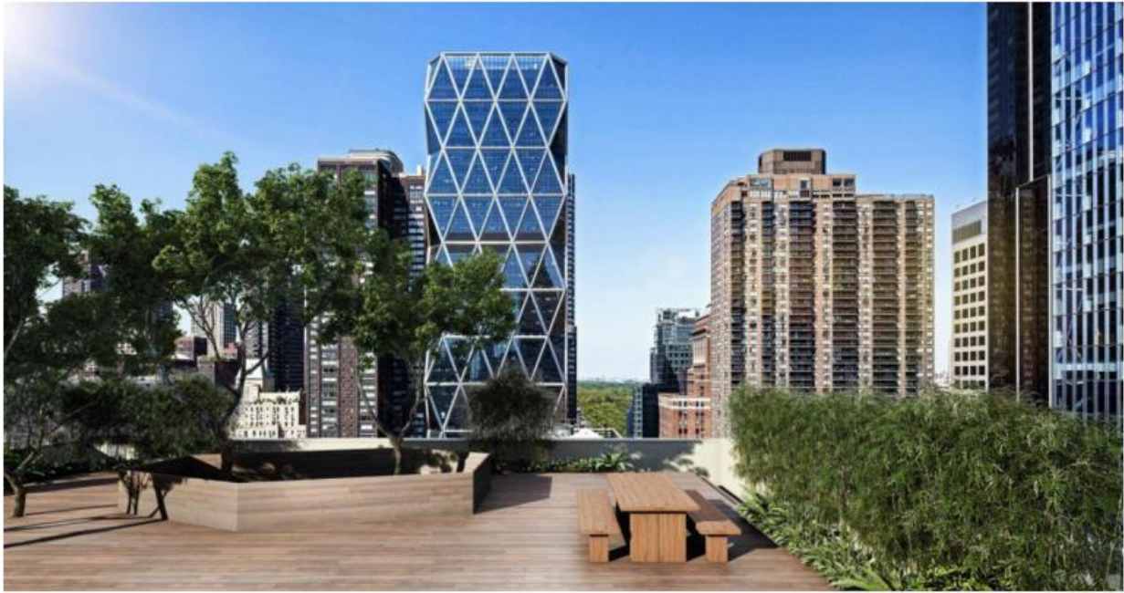
Rooftop terrace at 301 West 53rd Street
